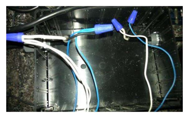
Put the faceplate on the box, pull the slack out of the power cords and snug down the cord connectors.
