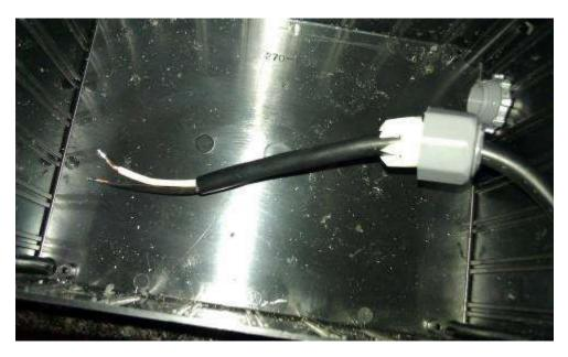
Insert through the connector, give yourself some slack, don't tighten the connector down yet.
