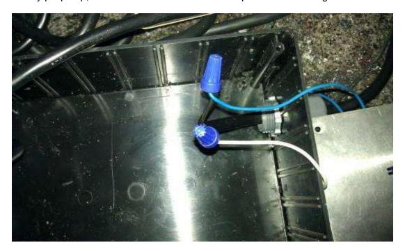
I used wirenuts to attach the nutrient pumps to the power cord coming in on that side. 2 pumps, same power, same outlet, both will activate at the same time. If I had another pump for an additive, I would wire that in to the same bundle.
