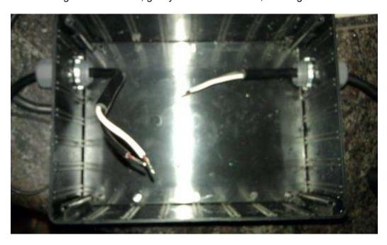
On my pH pump, I used wirenuts to connect to the power cord coming in from that side.
