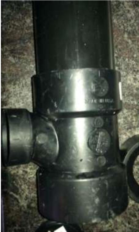
Glue in the reducer into the open end of the sanitary Tee.
